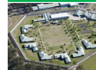
Outer Metropolitan Multipurpose Correctional Centre (OMMPCC), Sydney
